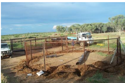
TANK FRAME WITH MESH WALL IN PLACE
